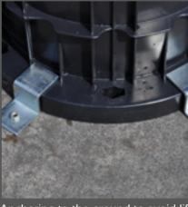
Anchoring to the ground to avoid lifting of the formwork is done using metal brackets or otherwise with timber.
