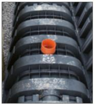
Upper side designed to insert a vent or inspection duct
