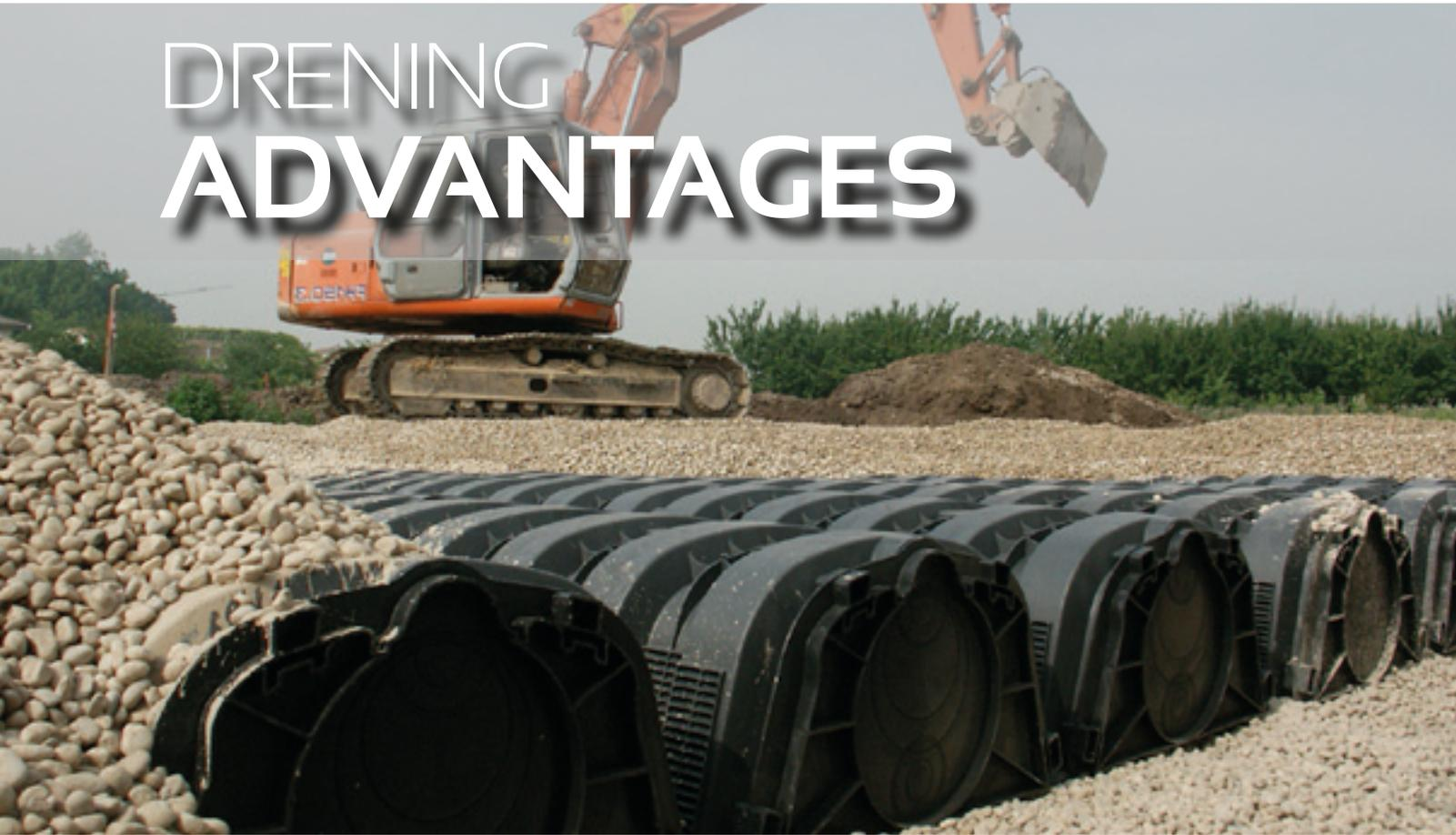
High resistance modular system for the creation of retention ponds and high capacity accumulation basins
