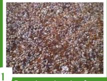
Excavation and creation of a draining layer made of gravel or lapillus (minimum 15-20 cm)
