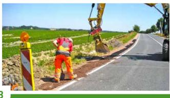
COVER UP TO THE EDGE OF GEOROAD WITH FINE-GRAINED. IT IS POSSIBLE TO COVER THE SURFACE WITH GRASS, TOO.
