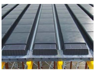
Once the supporting system is built (props+ yellow beams), place the beam elements made of ABS that create a regular support base for the domes.
