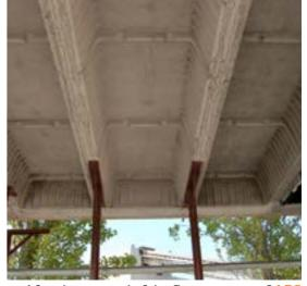
After the removal of the first two rows of ABS beams, it is possible to remove SKYRAIL and SKYBLOCK domes. When this operation is completed, the system should be shored again, in order to keep the shoring until 28 days after the concrete maturation.
